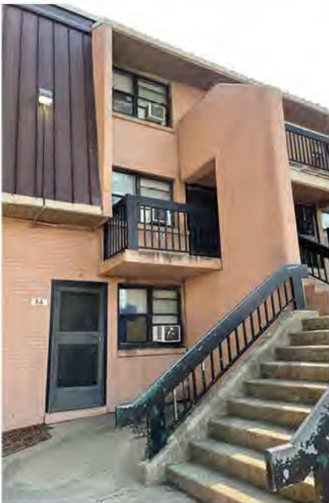
Residents at Gilpin Court must use window AC units, as the community is not equipped with central air.
