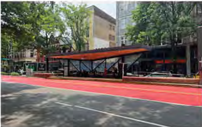
Pulse bus lane on Broad Street (City of Richmond)
