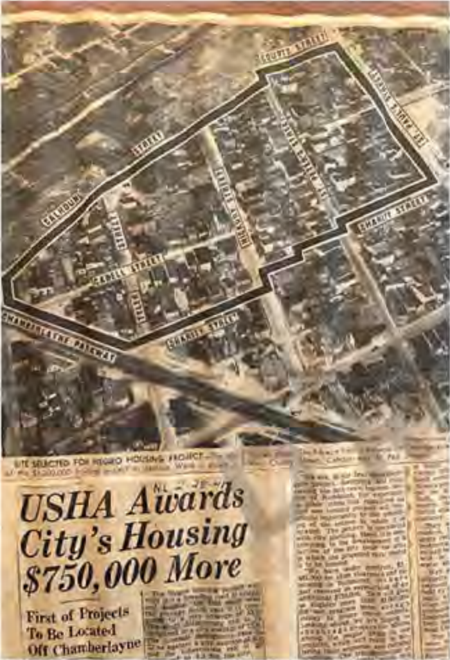
1941 news article announcing additional funds for the Gilpin construction
