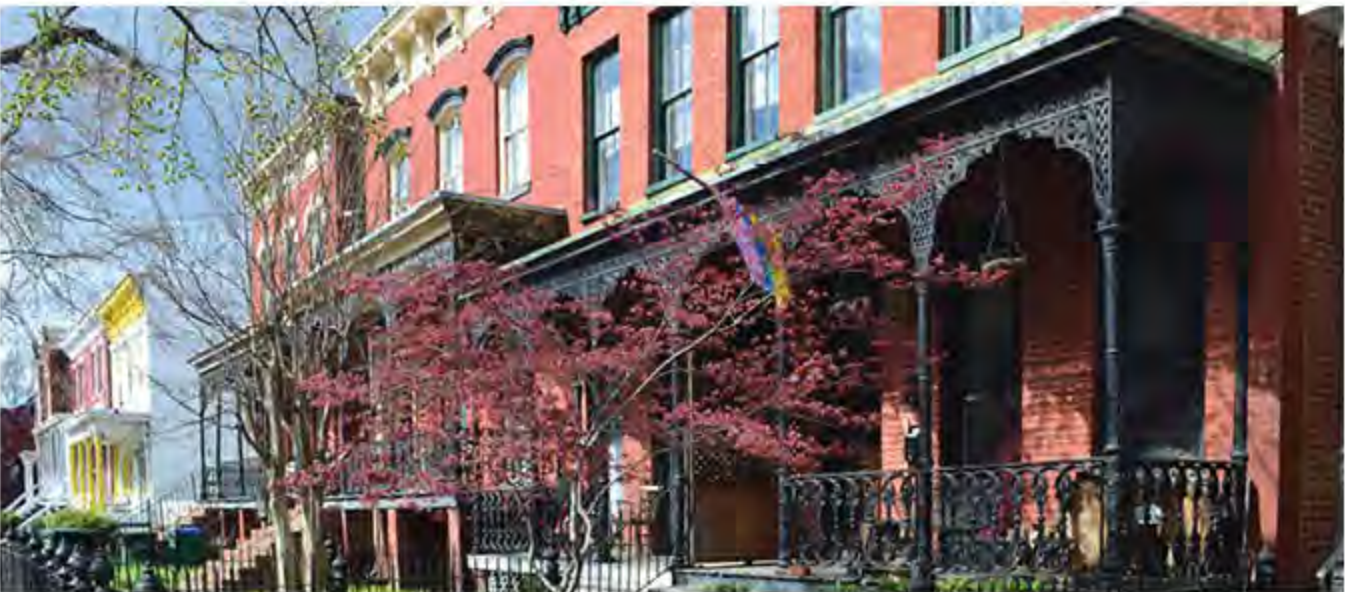
Jackson Ward row houses (Source: Virginia DHR, Calder Loth, 2019)
