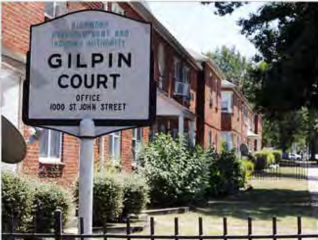
Gilpin Court Apartments
